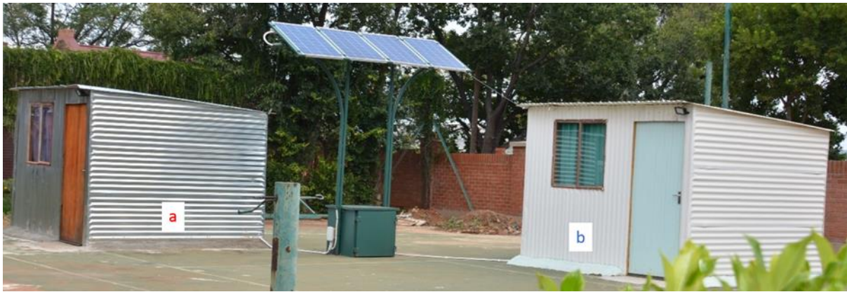
Figure 3: Experimental structures: a) uncoated (control) and b) coated.
