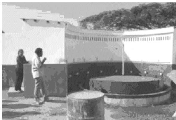
Figure 2: The biogas digester connected to flushing toilets at Myeka High School
