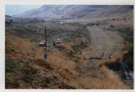
Figure 9: Single Wire Earth Return Transmission line
